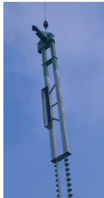
Attaching the upper part of a 30-metre elevator
